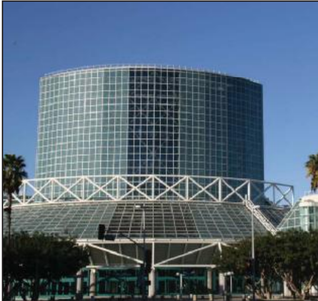
Los Angeles Convention Center - South Hall Tower
